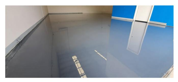
This is probably among the first impressions when epoxy flooring is brought up. Epoxy has a smooth and highly reflective surface, making it look slippery. In spite of that, epoxy is far from being slippery. It is actually **skid-resistant**, and you could opt for additional anti-slip features if you want. Likewise, you could add raised bumps for additional user safety.
