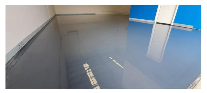
This is probably among the first impressions when epoxy flooring is brought up. Epoxy has a smooth and highly reflective surface, making it look slippery. In spite of that, epoxy is far from being slippery. It is actually **skidresistant**, and you could opt for additional anti-slip features if you want. Likewise, you could add raised bumps for additional user safety.
