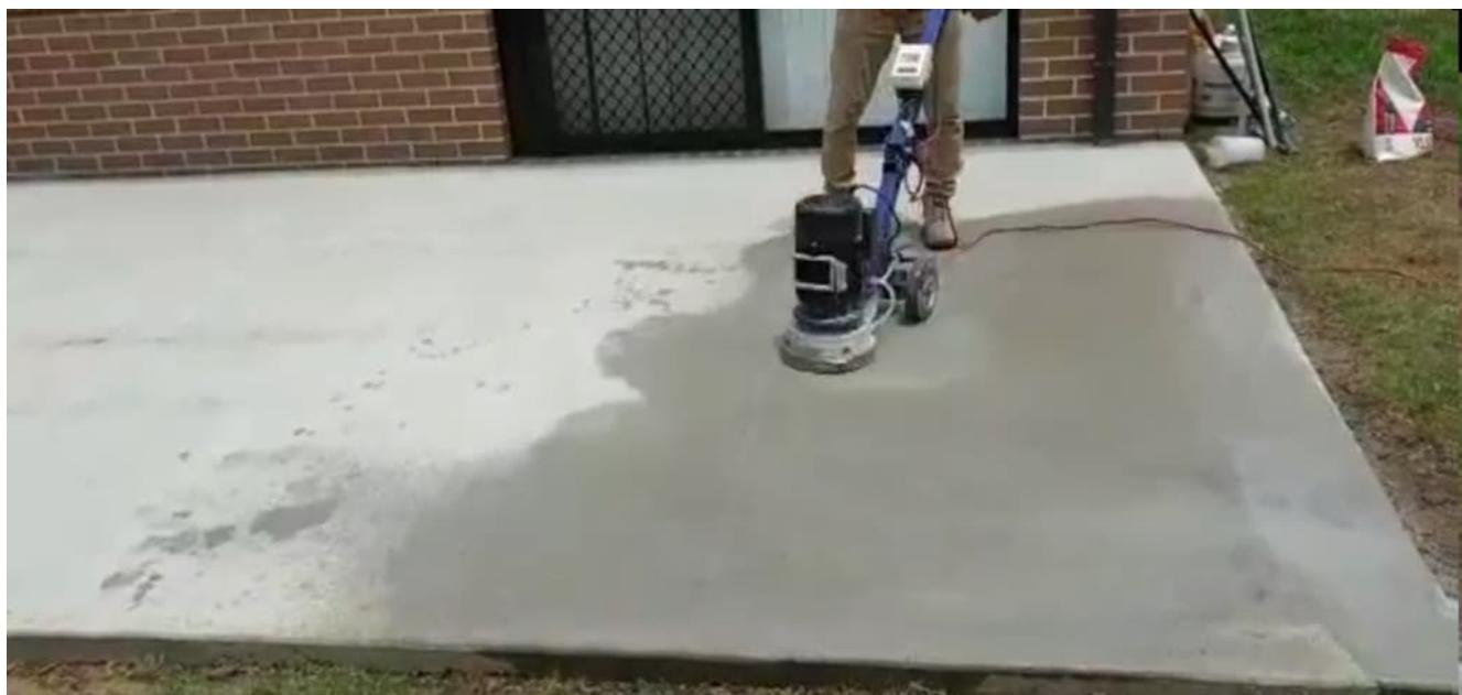
The concrete resurfacing process includes **cleaning**, **repairing**, and **overlaying** the floor with a new surface adding life to the aged concrete floor.
