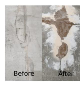
Self Leveling Epoxy can be applied over cracked concrete floors to create a durable and low maintenance flooring surface. This epoxy flooring can be ideally used over old, cracked and damaged concrete floors to create a smooth and seamless surface.
