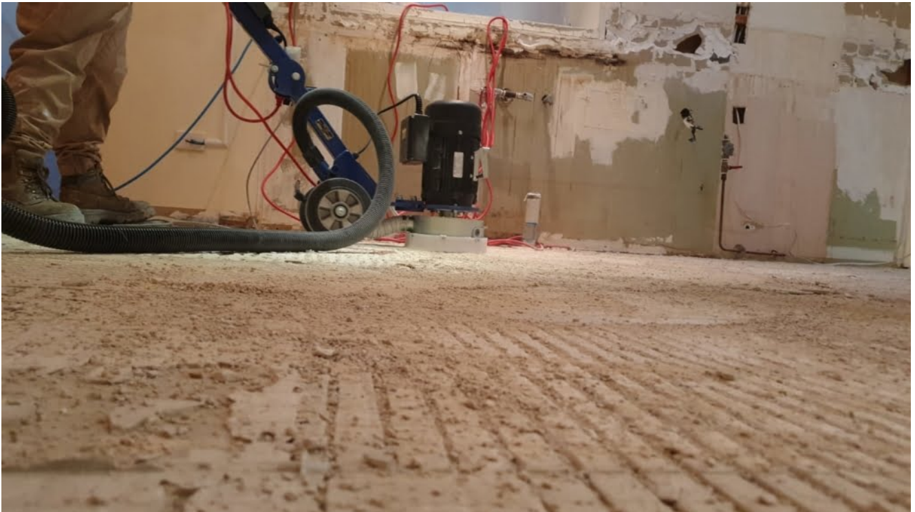
Tile Glue Removal Process and Machine
