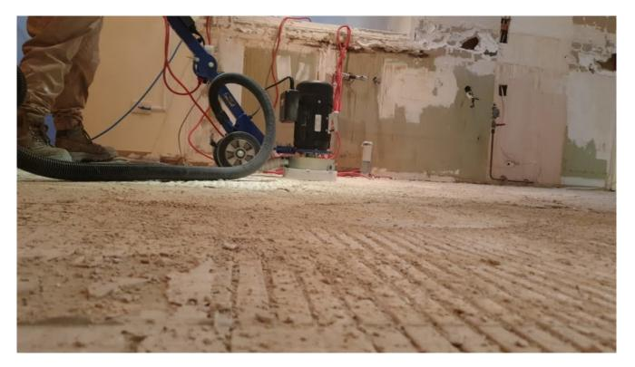
It is important to make sure that the base is clean to avoid a distorted result. Generally, a primer coat is applied to help the epoxy adhere to the floor. Then, the epoxy floor coating is applied using a different method based on the finish you choose.
